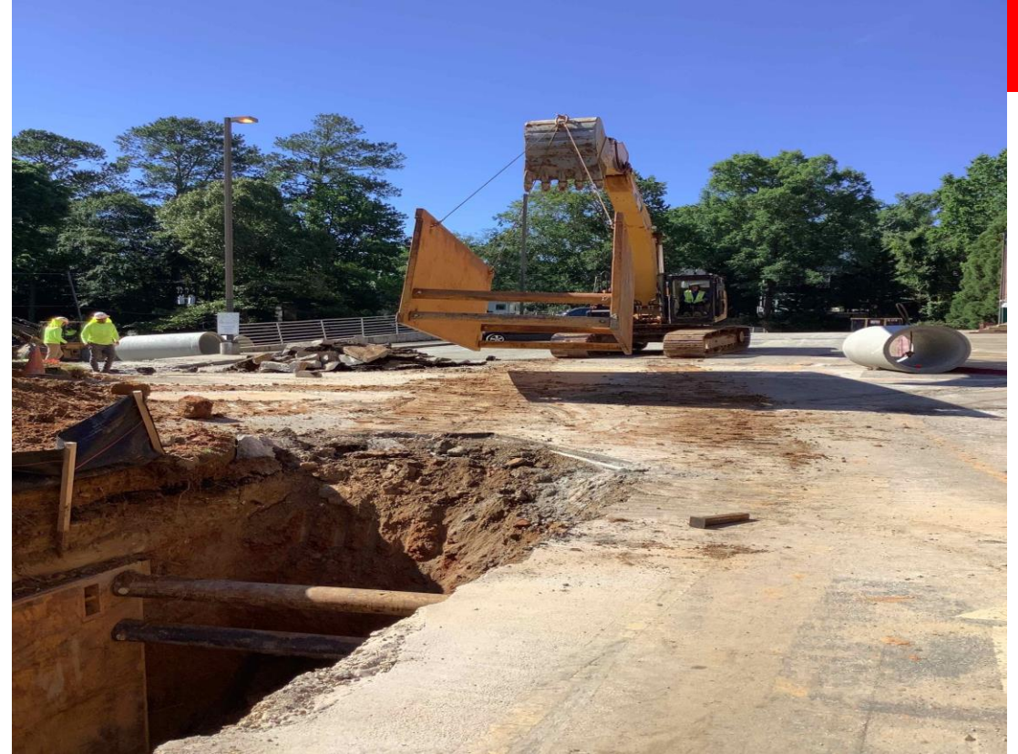
Storm drainage installation
