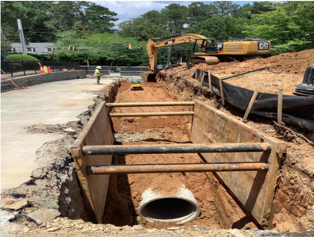
Storm drainage installation
