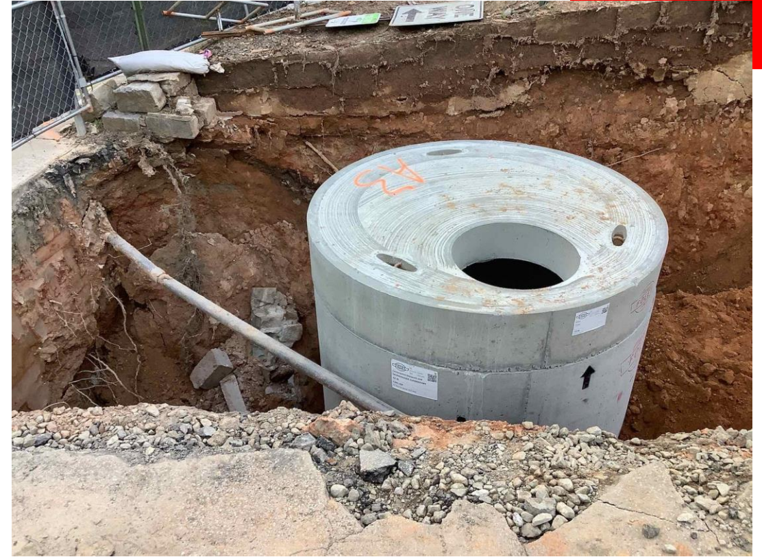
Storm structure installation
